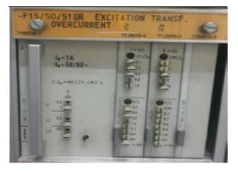
In Unit 7 there were individual relays for every protection. Trip output from these relays were extended to following locations through Trip Matrix (Refer Fig 2):
